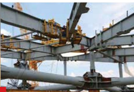
Multipoint system of lifting and lowering roof's frame "Spartak" stadium in Moscow, "Ruby" in Kazan and "Fischt" in Sochi.
