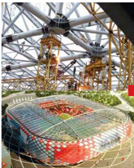
Multipoint system of lifting and lowering roof's frame "Spartak" stadium in Moscow, "Ruby" in Kazan and "Fischt" in Sochi.
