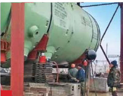
System for simultaneous lifting of the object for assembling the reactor plant of nuclear power station WWER – 1000, Volgondsk.
