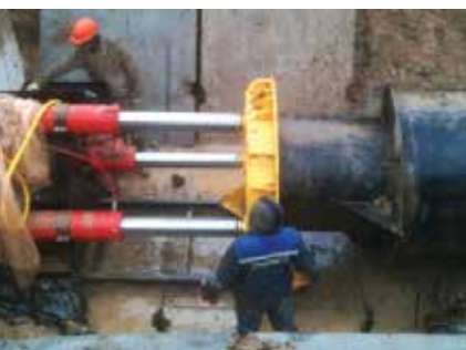
Trenchless pipes laying system UBPT «Horizon» for a governmental project «Oil pipeline «Easten Siberia–Pacific»
