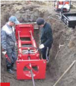
Equipment of a ground puncture – 25U UPG «Arrow» for trenchless installation of underground utilities. Manufacturing and supplying it to companies specializing in the laying of utilities.
